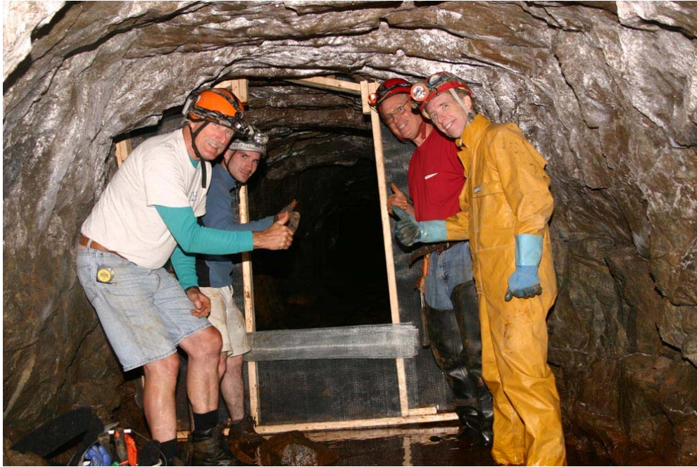
Fahnestock Mine bat gate construction w/DEC
