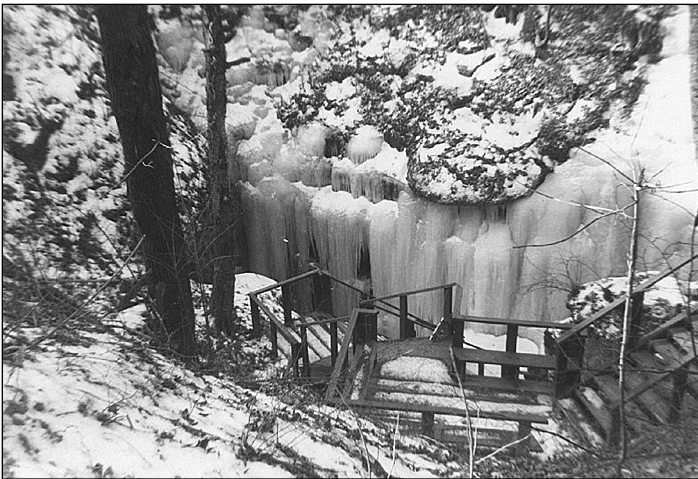
Stairs remaining from the commercial operation at the Knox Cave entrance (1969). Photo by Art Palmer.
